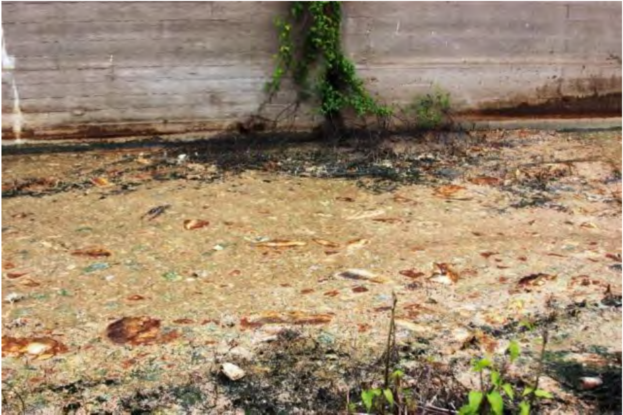
Figure 4.4. Decomposed dead carp and buffalo below the Morganza Spillway structure.
